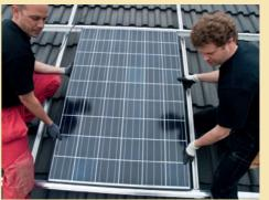
All cables are laid in parallel to the installed rails. Now the modules can be inserted. The modules are held in place by gravity and must not be fixed in place by screws.
