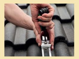
The horizontal TS insertion profiles are affixed using the connecting element SafeClick SC.
