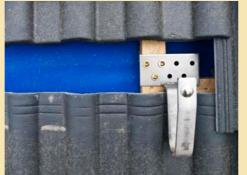
Depending on the type of roof, there are different ways of affixing the installation system to the roof: On pitched roofs the systems are installed with roof hooks, on trapezoidal and cement asbestos roofs with hanger bolts, on flat roofs either with gravel-bordered Renosol trapezoidal plates or with hanger bolts and building exterior systems are directly screwed into the building exterior.
